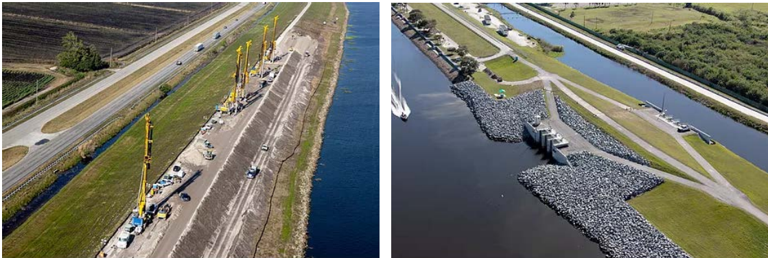
Herbert Hoover Dike (Photo Credits: USACE)
