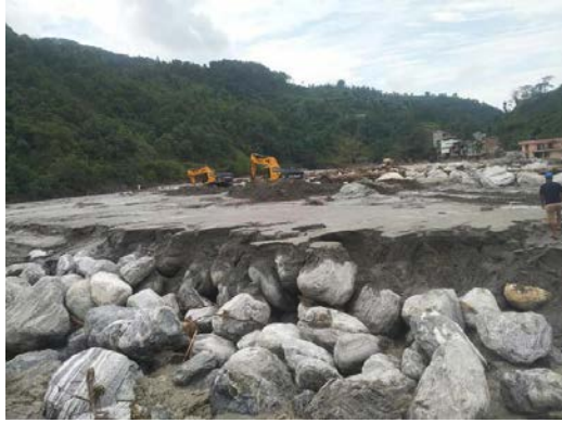
Excavators are working to re-channelize the Melamchi River in the previous course (Photo Credit: JB Karki)
