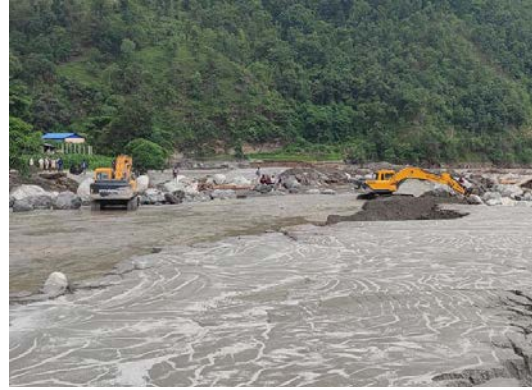
Excavators are working to re-channelize the Melamchi River in the previous course (Photo Credit: JB Karki)
