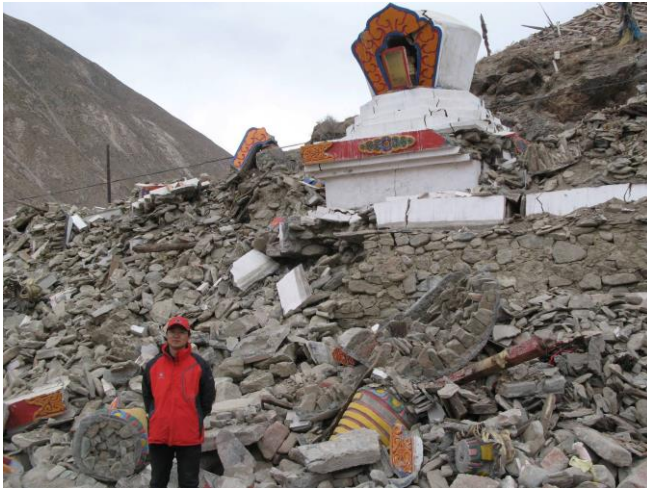
At the Yushu earthquake site with an altitude of 4200m
