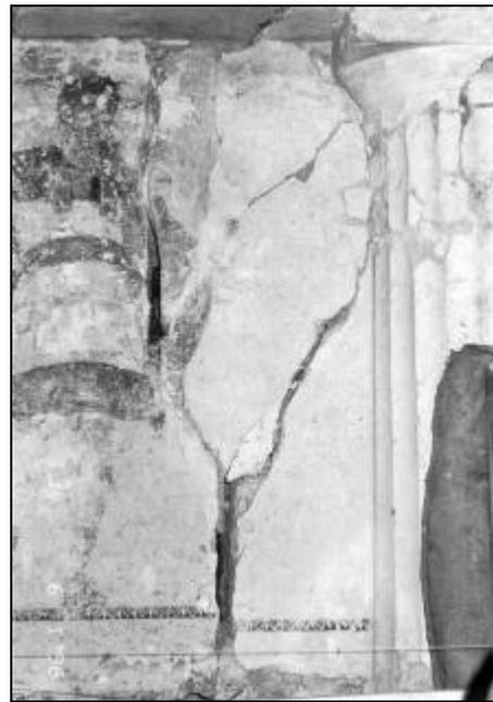
Figure 3: Krisis Tomb. The differential settlement caused failures and displacements on the front wall.
