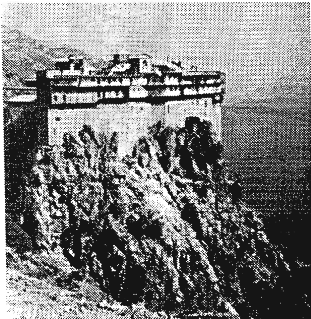
Fig. 2 - The rockmass where the monastery is constructed.
