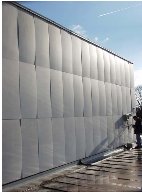
Figure 9. Facade clad with Carrara marble on a building in Göttingen, Germany
