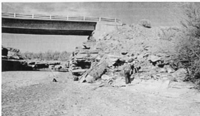
Left abutment of State Highway 262 bridge across Montezuma Creek in San Juan County, UT; evaluated as part of NCHRP rock scour study.
