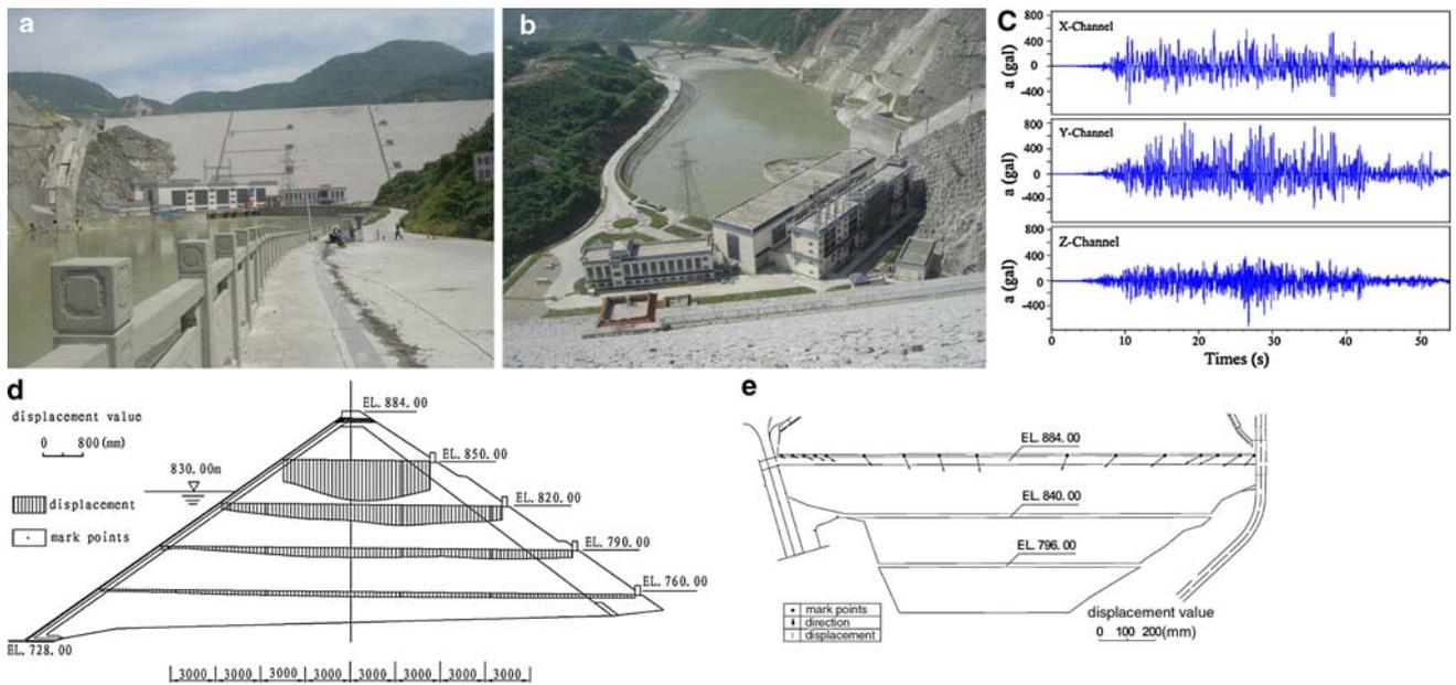
Fig. 10 Seismic behavior of Zipingpo dam in the Wenchuan earthquake. a Zipingpo dam, b Power house, c Seismic record (acceleration), d Vertical subsidence of dam top, e Horizontal displacement of dam top
