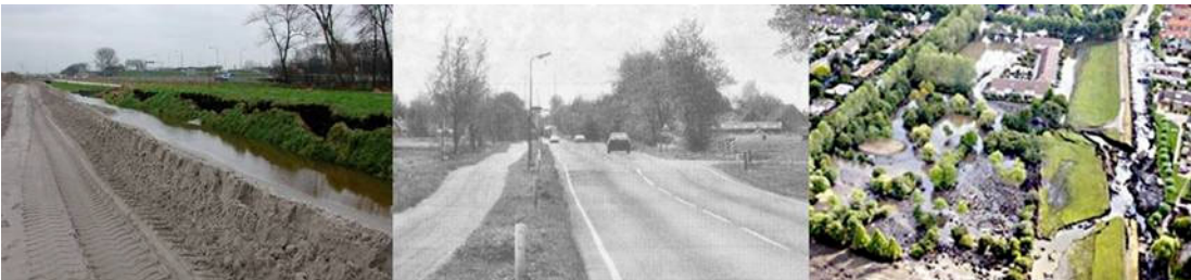
Figure 2. Squeezing of soft layers revealed during widening of a motorway (left). An “inverse” landscape (middle). Dike failure during a dry summer (right, from van Baars, 2005).
