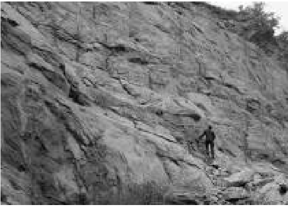
Figure 1. block structure gneiss
