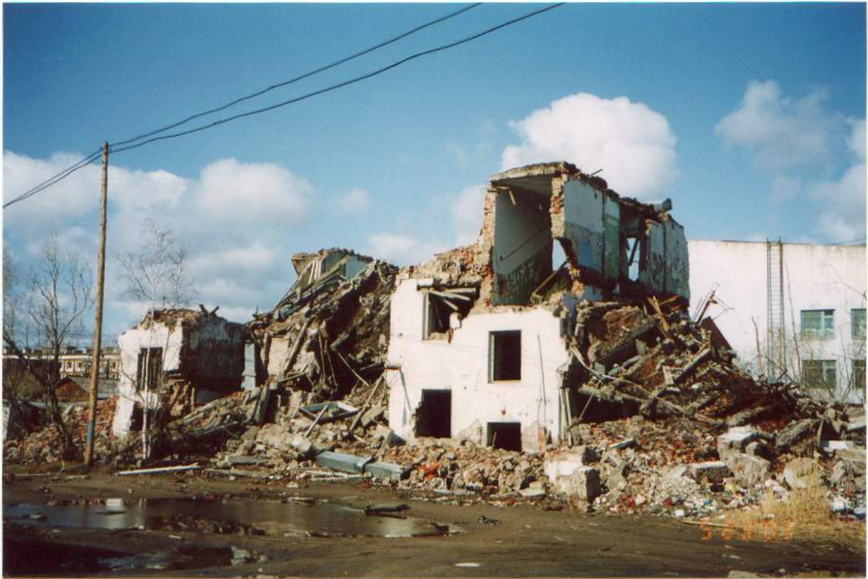
Figure 2. Destruction of buildings in Yakutsk
