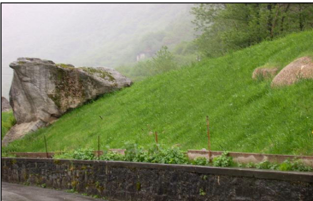
Figure 6. Lodrino (Canton Ticino), “Artificial loam” obtained from a similar bioremediation process a number of months after seeding (Fornaro et al. 2003).
