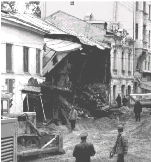
Figure 1. Destruction of building caused by suffosional collapse sink formation in Moscow in 1998
