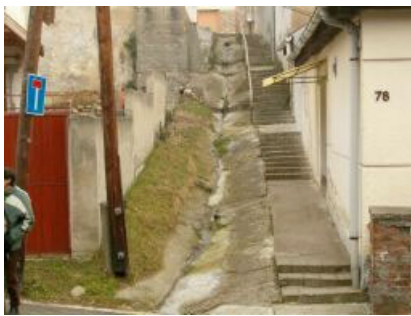
Figure 5. Precipitation drainage ditch (Pécs)
