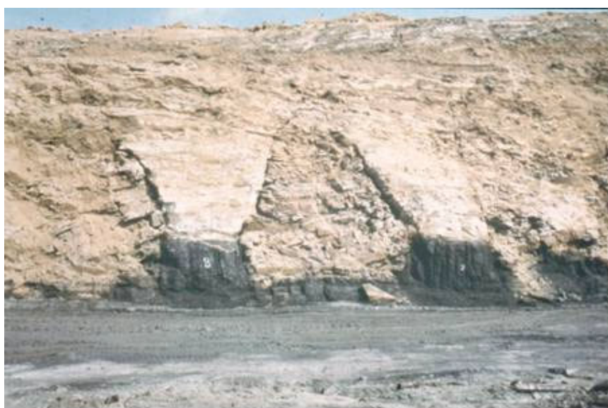
Figure 6. Crown hole collapse uncovered during opencast excavations (Photo courtesy Prof Paul Younger)
