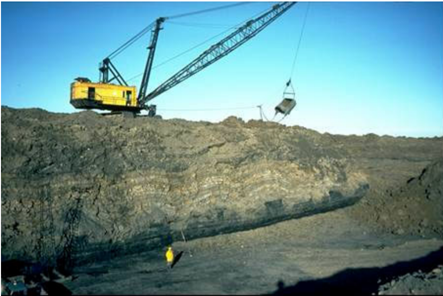
Figure 7. Creep deformation over pillars uncovered during opencast excavations at Langley site, Co Durham
