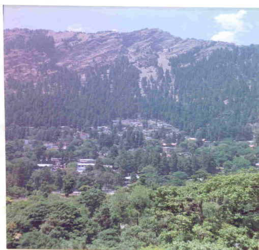
Figure 1. Naina peak slide zone and development of debris cone. Urbanization below is at risk .
