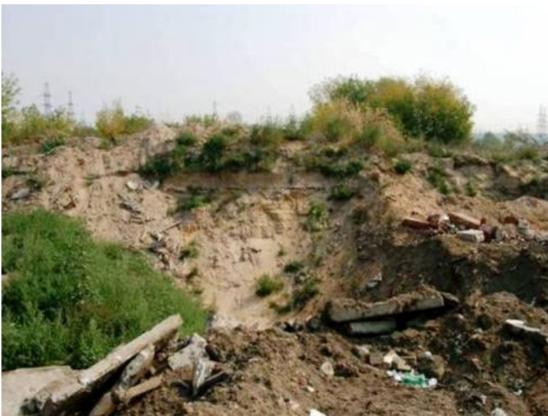
Figure 2. The fill soils
