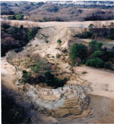
Figure 3. Picture of the Takarazuka landslide that followed the Great Hanshin earthquake of 1995.
