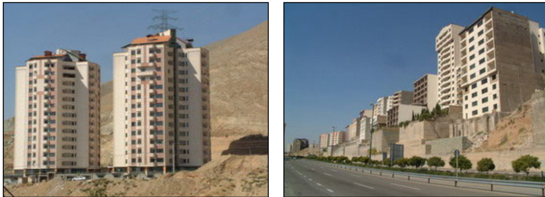
Figure 4. Construction of new apartments blocks along the trend of Tehran's main faults.
